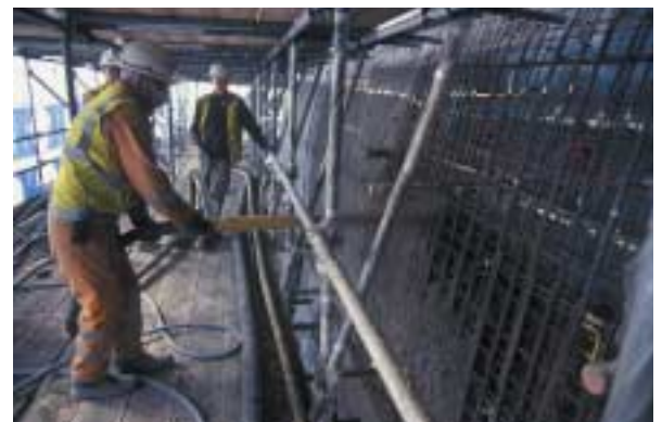
11. Spraying the substrate on site.
