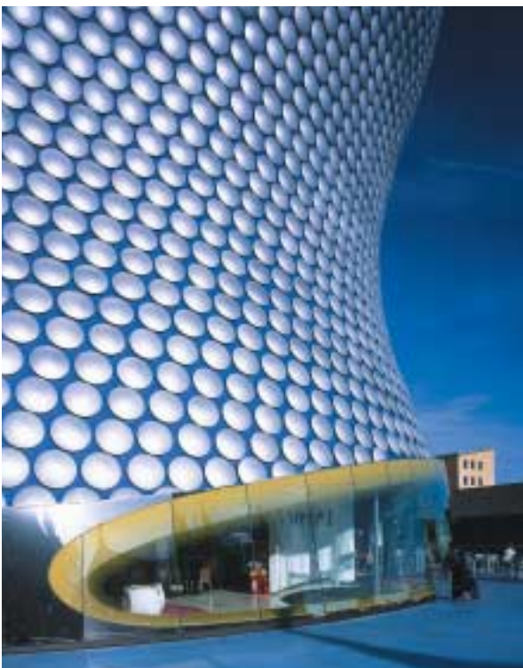
13. Glazing at terrace-level entrance.
