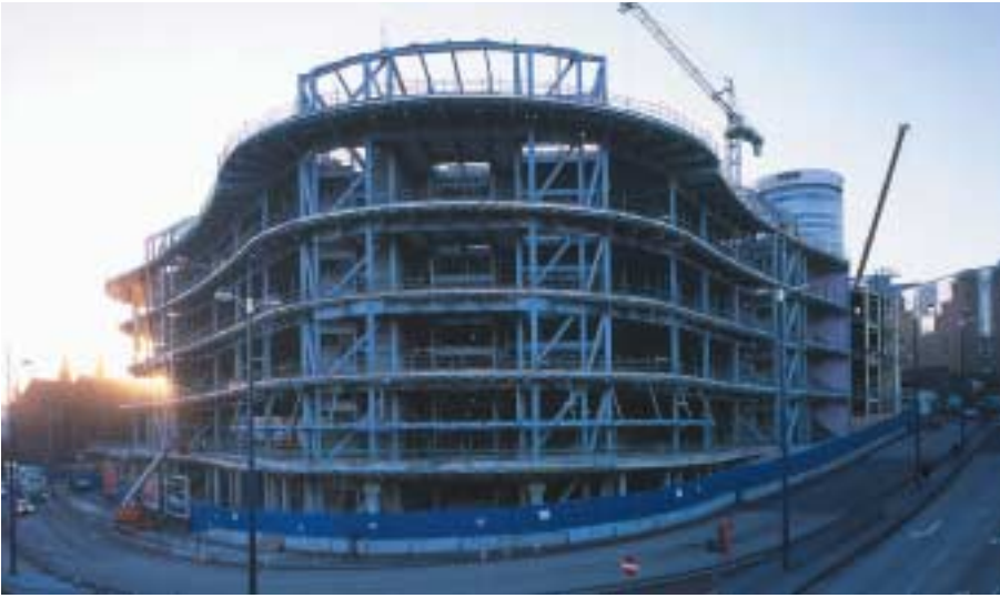
8. External view of completed frame.
