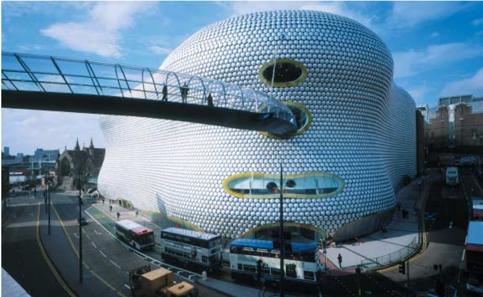
22. The completed Selfridges store and its link bridge in their Birmingham setting.
